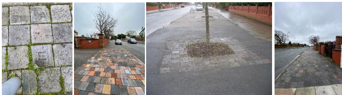
Southport paviers survivors in Hesketh Road, the most colourful section is in the kerb drive of No. 40 Hesketh Road
