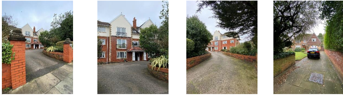
From left to right No. 12 Hesketh Road and No. 10a Hesketh Road
