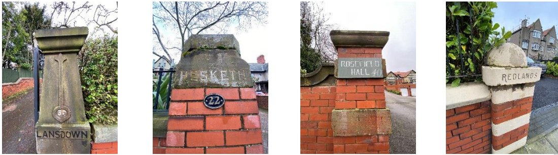
Examples of gate piers.
